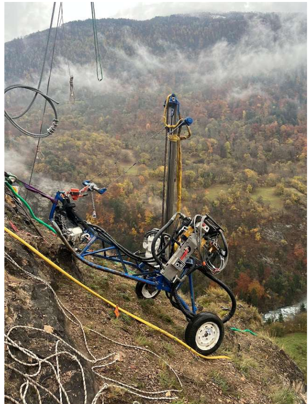
Figure 9 . Atelier de forage NGE FONDATIONS
