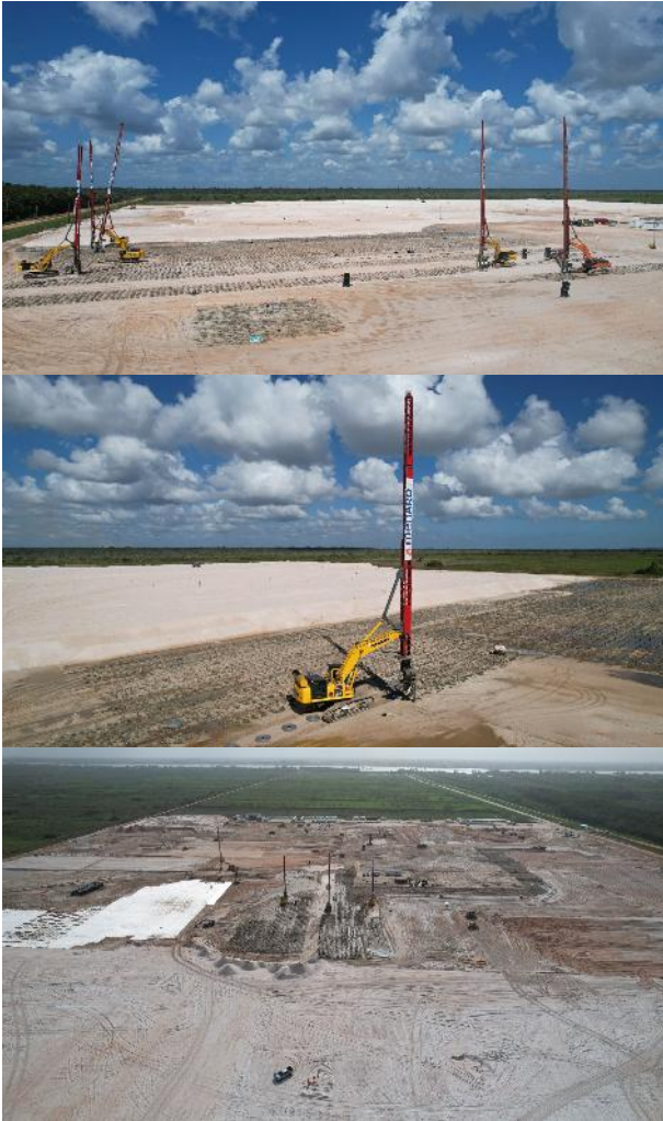
Figure 14. Installation des drains
